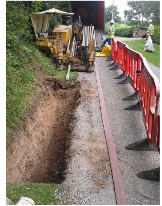
Image 2 : Typical Drilling Rig and Launch Pit
