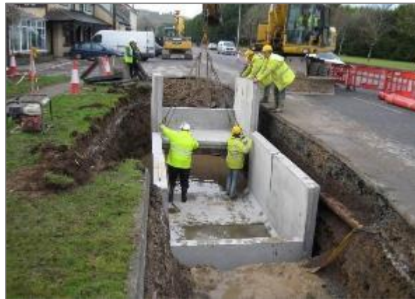
Figure 10 - Typical joint bay under construction (pre-cast)
