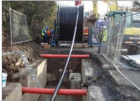
Figure 11 - HV cable pulling procedure (Typical drum set-up)
