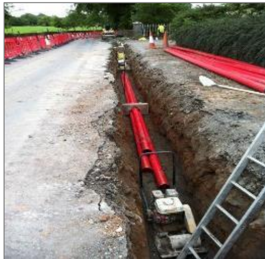
Figure 2 Typical 110kV Underground Duct Installation
